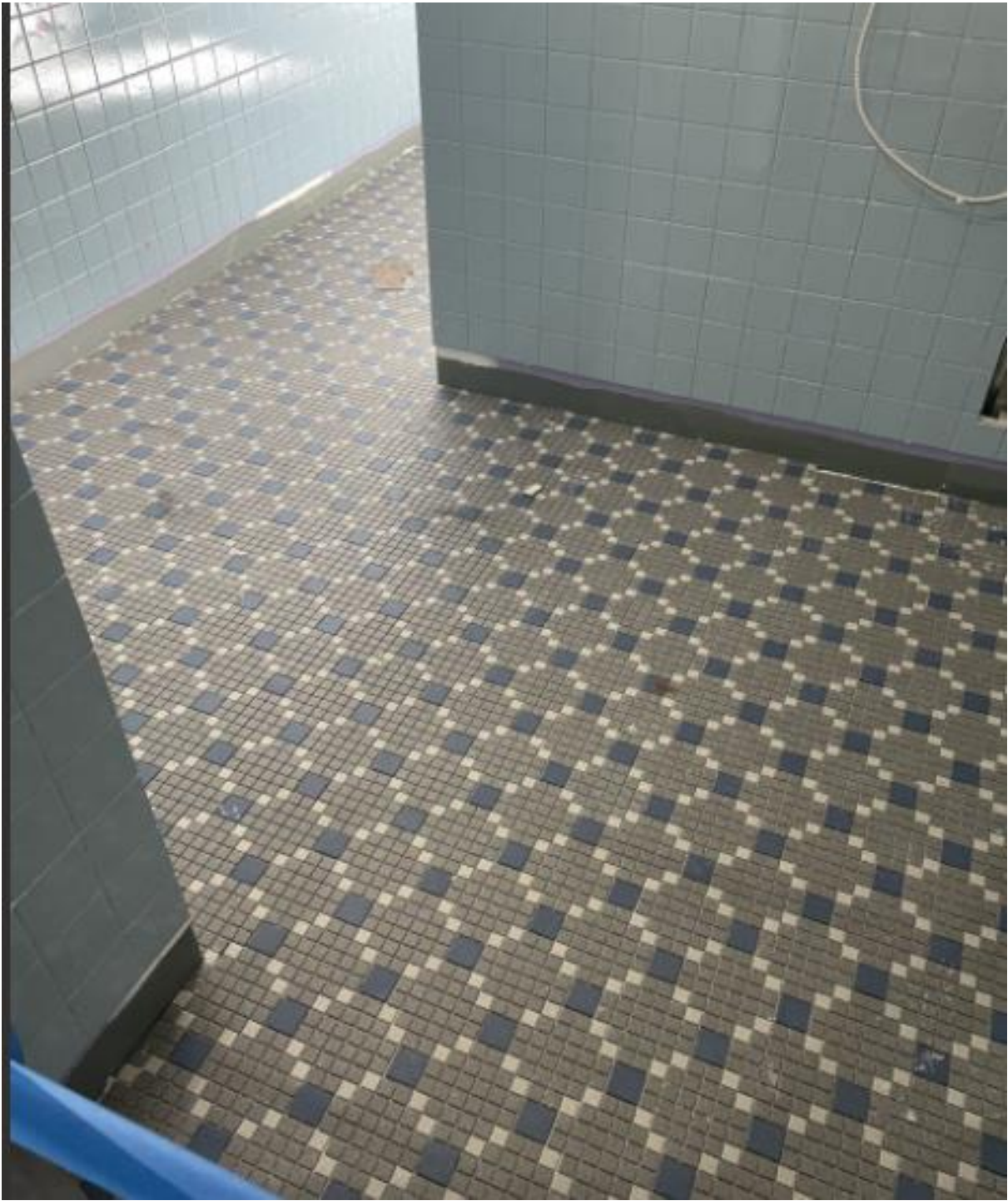
Our student bathroom walls and floors are being tiled.
